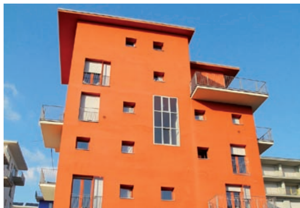
▲ Field tests of residential heat pumps show good performance and considerable CO 2 emissions reduction.
