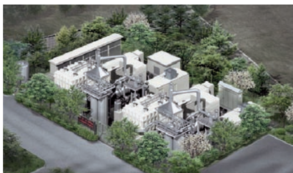
▲ This molten carbonate fuel cell plant produces 2.4 MW of electricity (Nowon, Korea).
