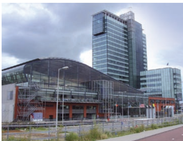
▲ Sustainable heating and cooling in the Oostelijke Handelskade complex (Netherlands).
