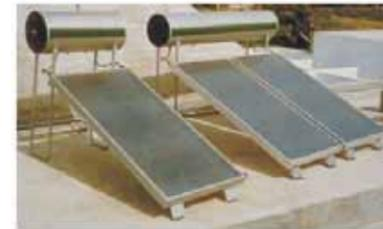
**Fig6: Compact type FPC based system**
