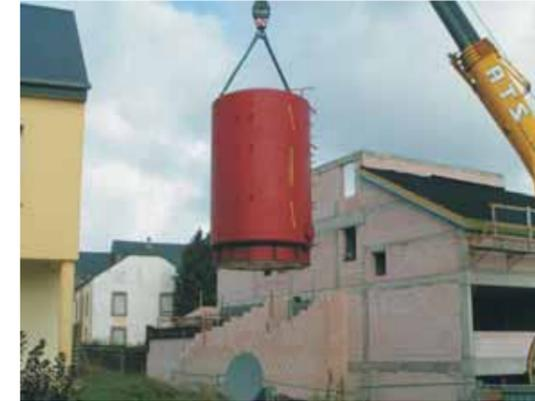
**Fig11: Installation of storage tank**
