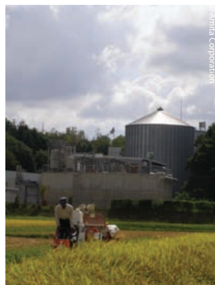
Paddy fields and biogas plant
