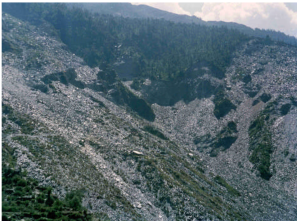
Fig.1: A View of Degraded Slope Due to Dumping of Slate Waste
