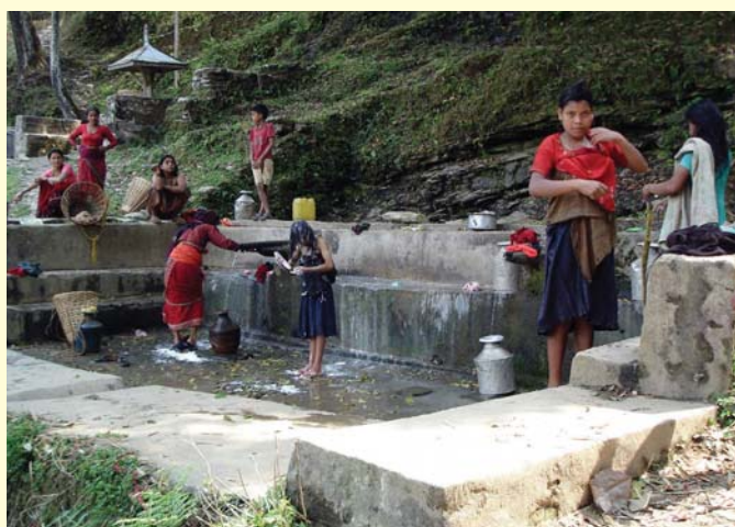
Community managed water pumping system
