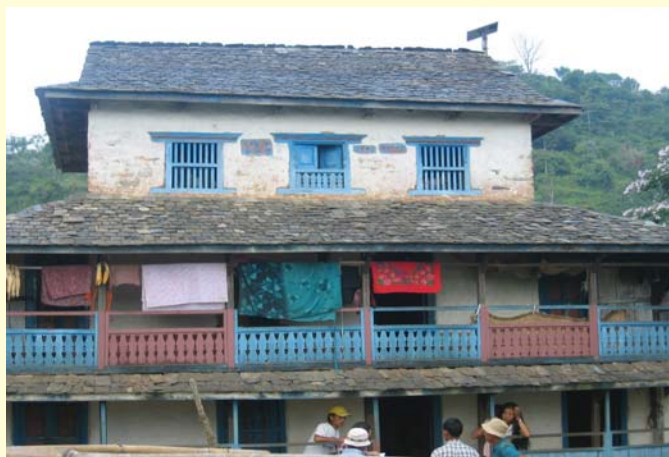
Solar Home System (SHS) Installed in Rural House
