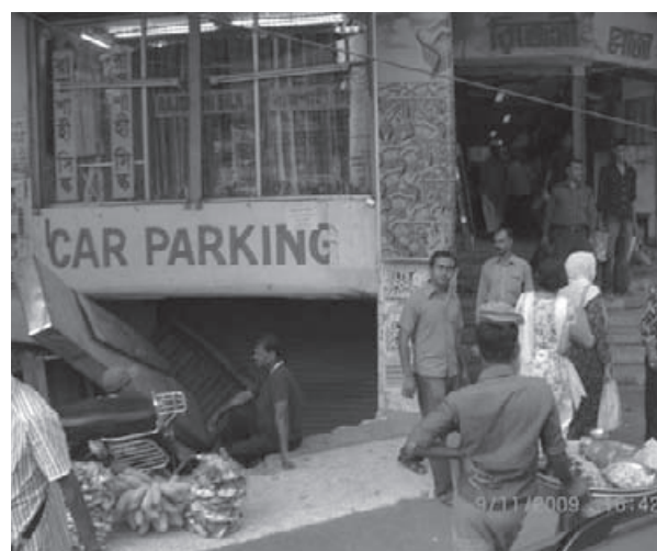
Basement in a commercial street in Dhaka signposted as "car parking" (but there are stairs, not a ramp, and this space had been used for shops before being demolished, presumably during an enforcement action)
