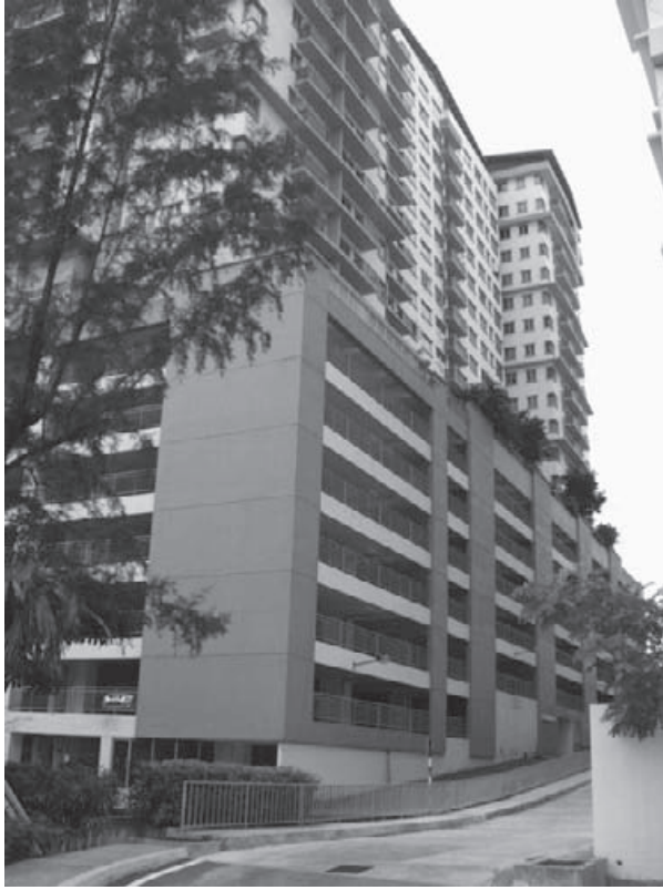
Parking floors in a residential condominium in Subang Jaya in Kuala Lumpur
