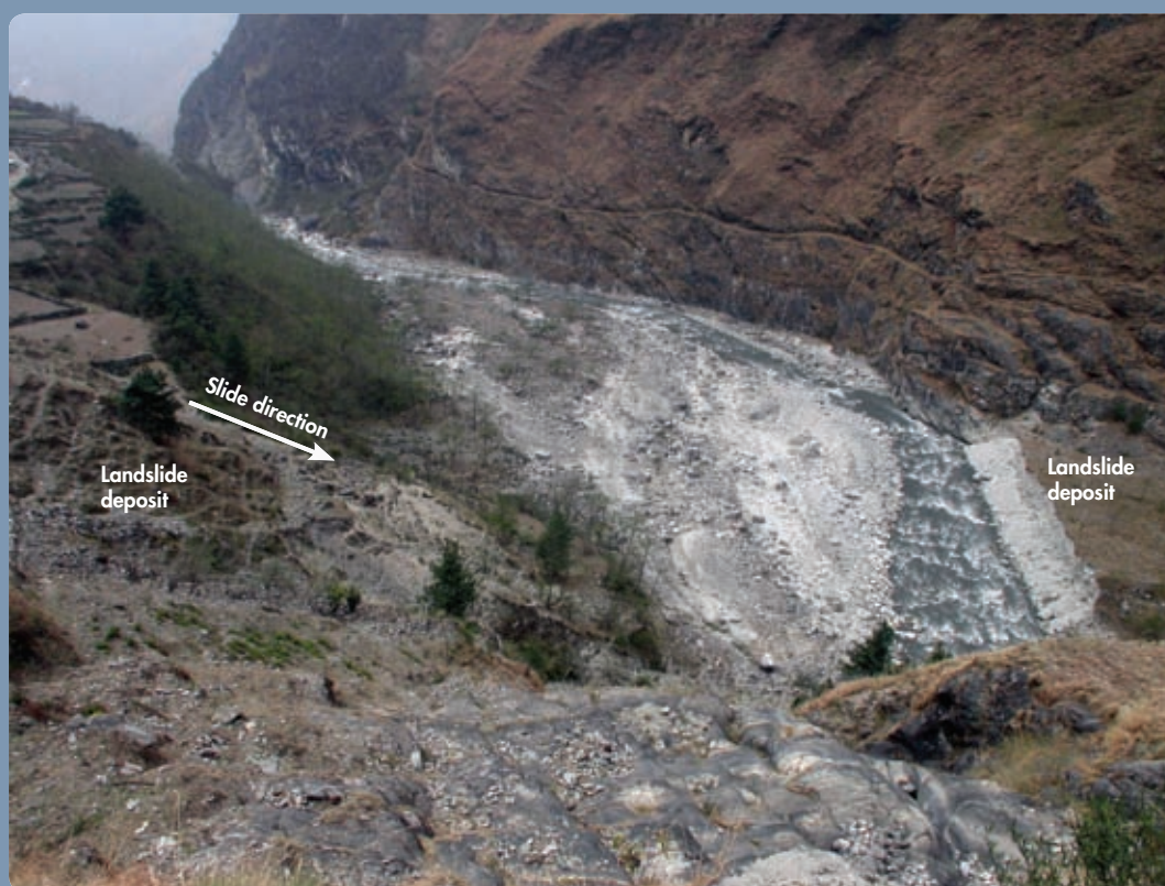
Figure 5: Breached landslide dam in the Kali Gandaki river at Thaple Pairo village
