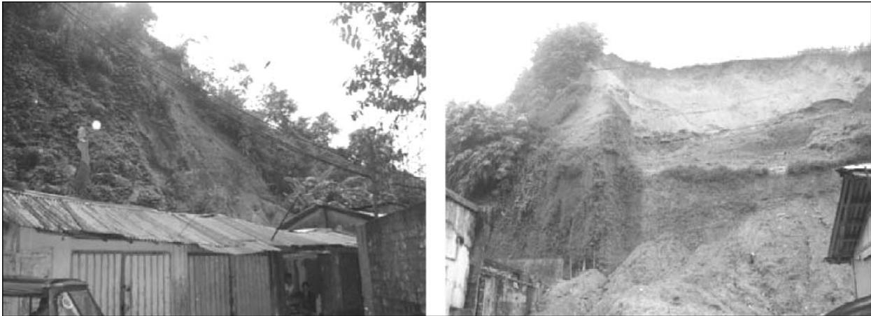
Figure 4: Showing the landslide happened due to hill cutting for construction purpose
