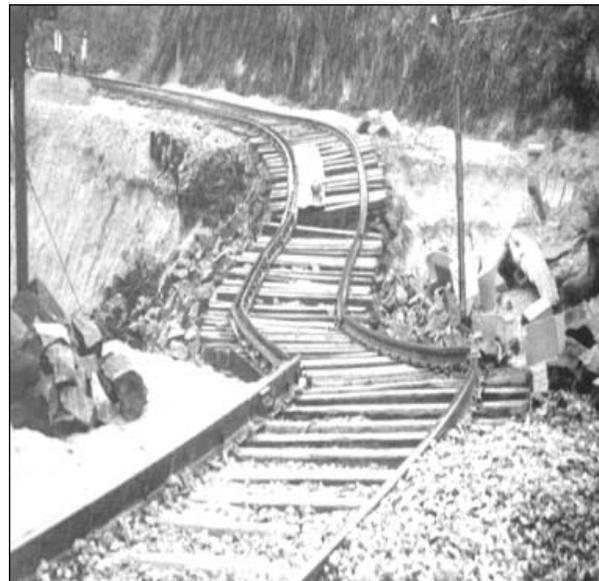
*Figure 14: The more than 100 year old Watawala Earthslide in Sri Lanka was completely controlled through use of innovative subsurface drainage technology. Despite this, no other SAARC country has used this technology to control similar landslides. (Courtesy: R. K. Bhandari)*
