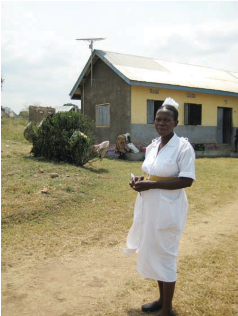
A health-care center powered by solar PV lighting in Uganda
