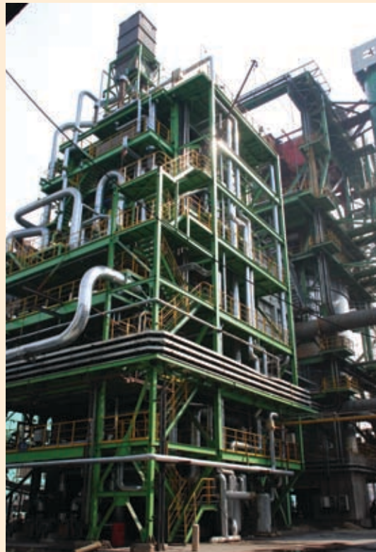
Baotou Iron and Steel Company plant, Inner Mongolia
