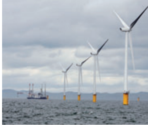
Robin Rigg offshore wind farm, UK. Photo: E.ON Climate & Renewables
