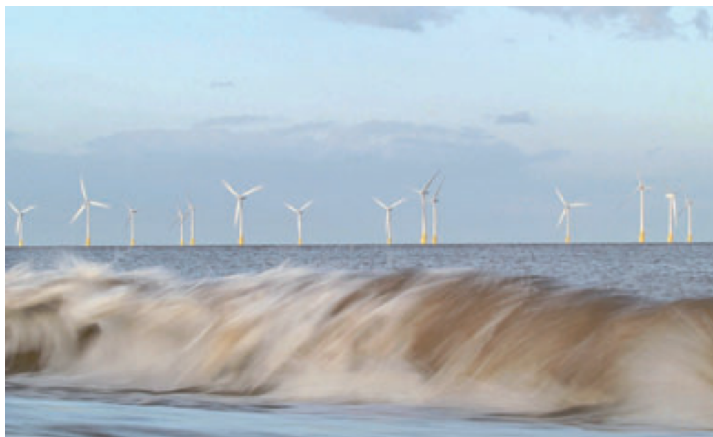
Scroby Sands offshore wind park, UK. Photo: E.ON Climate & Renewables
