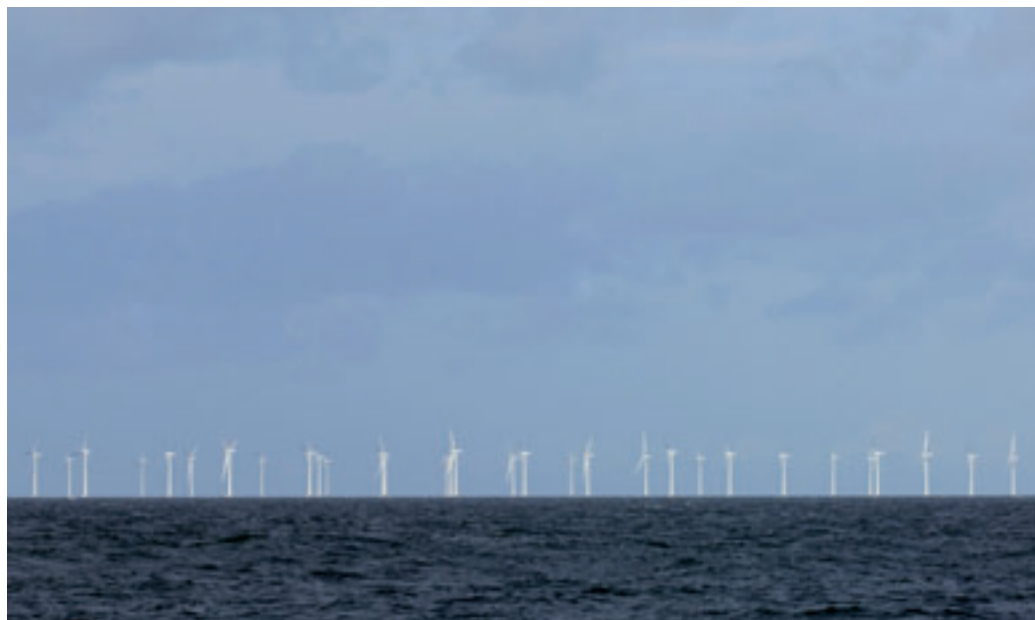
Lillgrund wind farm in Sweden. Photo: Jerker Lokrantz
