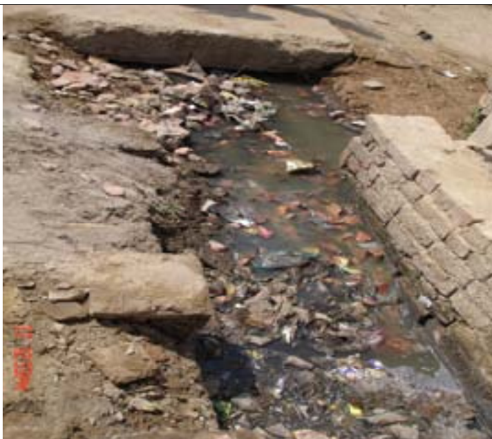
Exhibit 4.1: Broken Storm Water Drains which helps in increasing Siltling and Seepage from the Surrounding Environment
