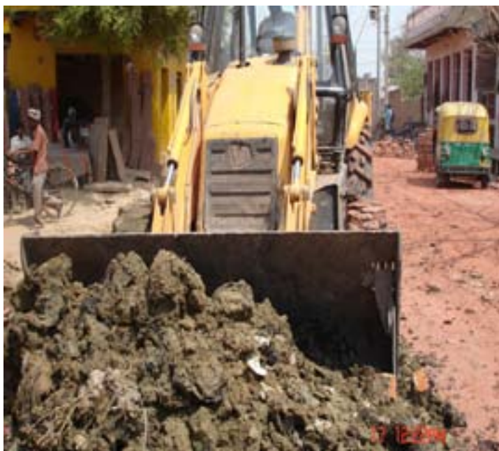
Exhibit 4.8: Excavated Silt and Sludge is dried on the Roads before removed through Excavator for Disposal into Low-Lying Area
