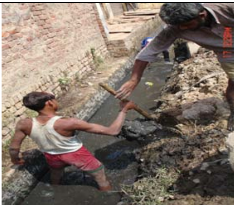
Exhibit 4.4: Sludge and Silt Removal from Storm Water Drains by Workers. Workers not protected while undertaking the task
