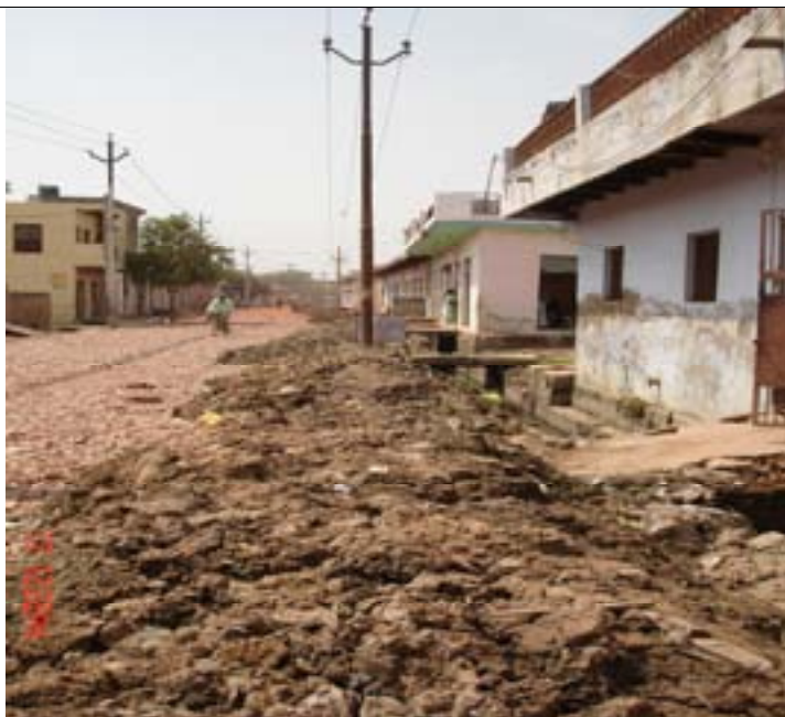
Exhibit 4.7: Excavated Silt Material in front of a House blocking entry to the House and reducing the Width of Road
