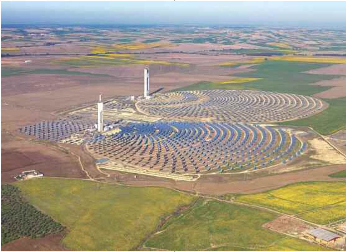
Solar energy towers in Seville, Spain.
