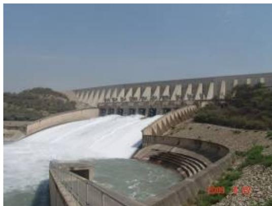
Since the reservoir capacity had reduced to 4.674 MAF from 5.88 MAF due to sediment deposition, raising of Mangla Dam by 30 ft. was taken in hand which has now completed. The Project will provide additional water storage of 2.88 MAF, increase water head by 30 ft and power generation of 644 GWh per annum and further flood alleviation.
