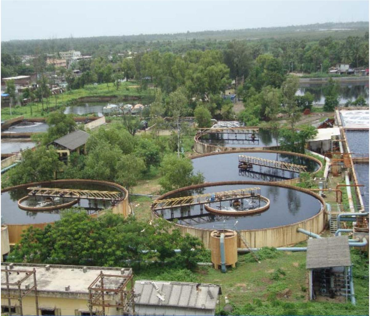
**A View of Activated sludge process under operation**
