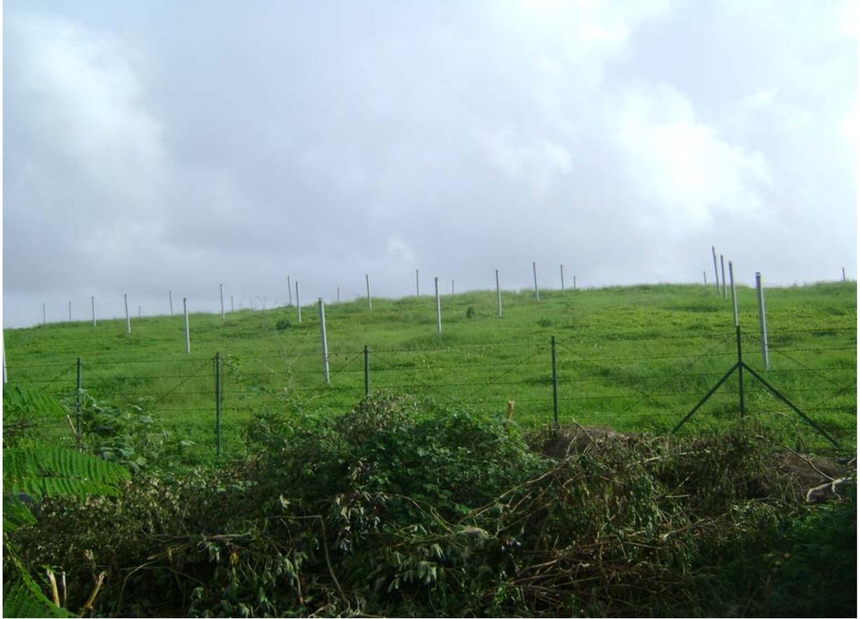
**Secured landfill site after encapsulation**
