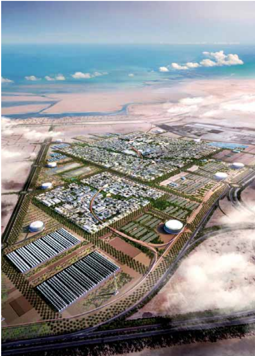
Aerial view of Masdar city once completed
